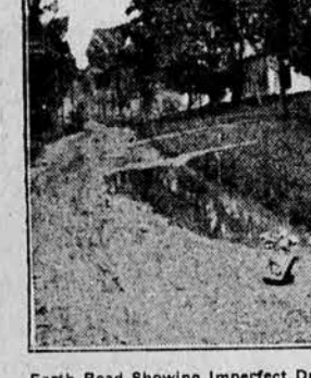
Earth Road Showing Imperfect Drainage.
