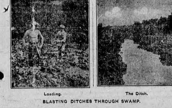
Loading. The Ditch. BLASTING DITCHES THROUGH SWAMP.
