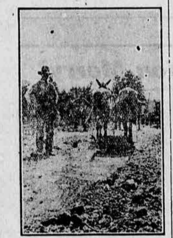
ROAD IN NORTH CAROLINA WORKED BY STAPOTE LADDER.
