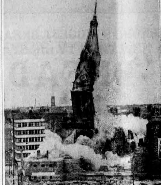
BERLIN COMMUNISTS BLOW UP CHURCH . . . The historic Georgian church, one of Berlin's most famous landmarks, was destroyed by the fire and explosives of World War II. The Communists, contrary to reports by engineers, termed it unsafe and destroyed it by dynamite. Protestant leaders protested, but the demolition squad destroyed it as Communist police and Russian soldiers cowed an indignant crowd of Berliners. The church was damaged by World War II bombs.
