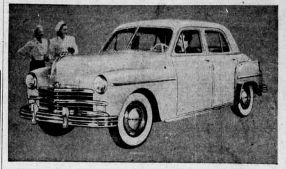
need hodies are lower and narrower, seats are wider and headroom greater. At the same time overall dimensions are reduced, but wheelbase has been lengthened to 118 inches and glass area is increased ower is raised to 97. Although fenders flow gracefully into the body they are detachable for ease in repair
