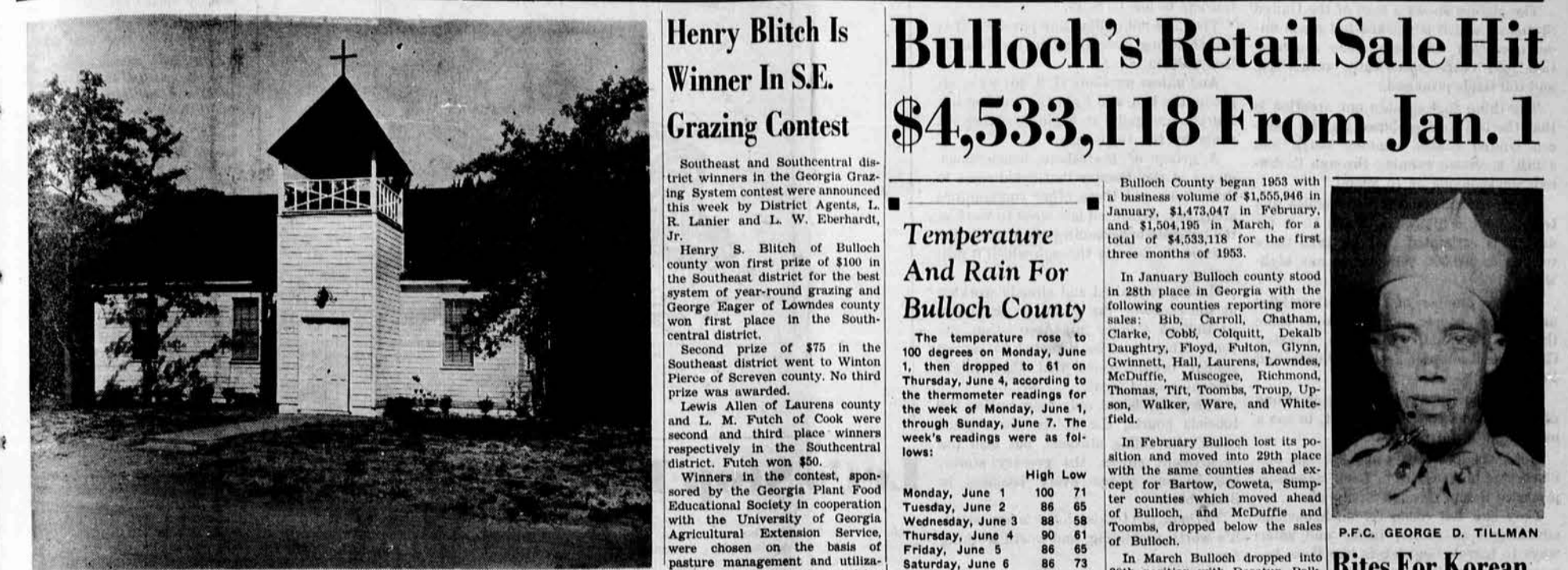
TRINITY EPISCOPAL CHURCH which was dedicated in special ceremonies on May 31, Trinity Sunday. The new church is located on Lee Street on U. S. Highway 80. Ernest Cannon was the contractor.
