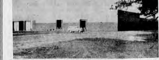
SOMETHING NEW IS ADDED—Here is the new section which was recently completed, increasing the floor space of the Rockwell plant here in Statesboro to 120,000 square feet.
