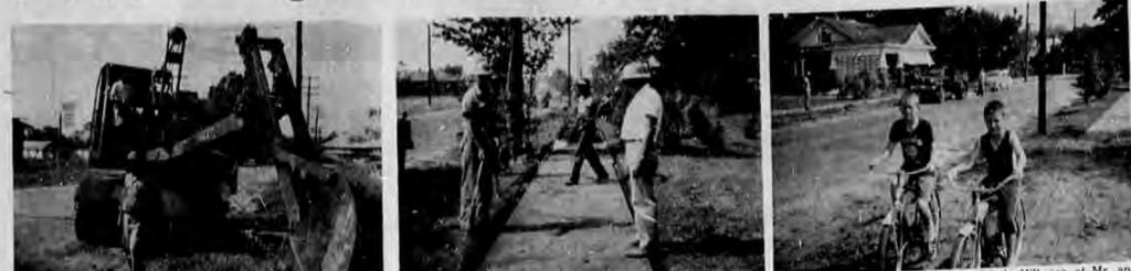
DEVOE DURDEN, drag line operator for the city waits for Homer Lanier, foreman, to give him the "go" sign to begin clearing for the new sidewalk construction on South Zetterower Avenue leading to the Recreation Swimming Pool and Park.
