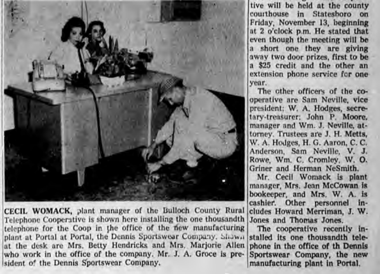
CECIL WOMACK, plant manager of the Bulloch County Rural Telephone Cooperative is shown here installing the one thousandth telephone for the Coop in the office of the new manufacturing plant at Portal at Portal, the Dennis Sportswear Company, which work in the office of the company. Mr. J. A. Groce is president of the Dennis Sportswear Company.
