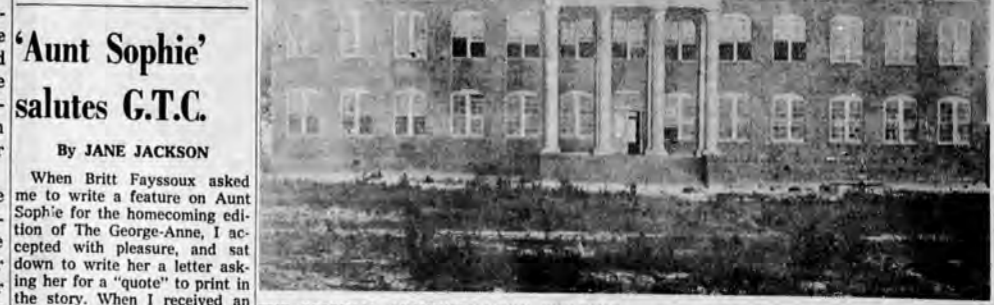
THE ORIGINAL ADMINISTRATION BUILDING , constructed at the beginning of the operation of the First District Agricultural and Mechanical school along with East and West Halls, at a cost of $45,000, has been renovated almost every year for the past fifty. Appropriations were granted for an auditorium to be annexed to the rear of this building during Guy H. Wells' presidency. The building is still used for the classroom space and offices of the dean, student guidance counselor, registrar, comptroller, and various professors. The water pump in the right front of the picture has been replaced by the water tank a little to the right of the center of the building.
