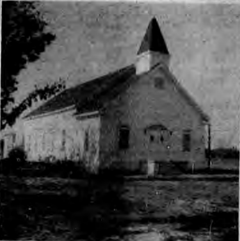
THE HARVILLE BAPTIST CHURCH, shown here, has recently completed a building program which included the renovating of the old sanctuary, and adding extra Sunday School rooms and additional space in the auditorium. The Rev. Inman Gerral is the pastor of the church and has served it since May, 1957. Mrs. Gerral is the former Miss Tomalee Alderman of Statesboro. They have four daughters.
