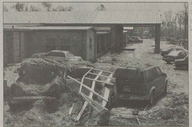
Steve Senne/Associated Press Mud and debris covers the perimeter of St. Rita's nursing home in Chalmette, La., Wednesday, Sept. 14, 2005. The owners of the home were charged with homicide for not evacuating the facility as Hurricane Katrina approached.
