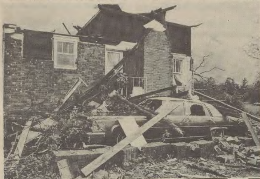
High winds destroyed 30 houses and 160 more were damaged.
