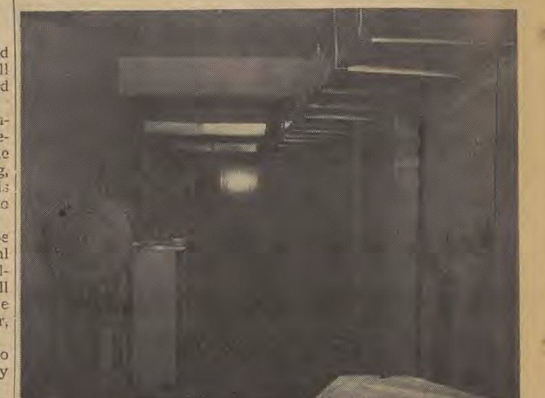
BASEMENT HERTY BUILDING — The above (pictures) the basement of the Herty Building as it now looks with the recent addition of classrooms and offices. The renovation is not expected to be completed for several weeks. However, classes are already being held in the new rooms.
