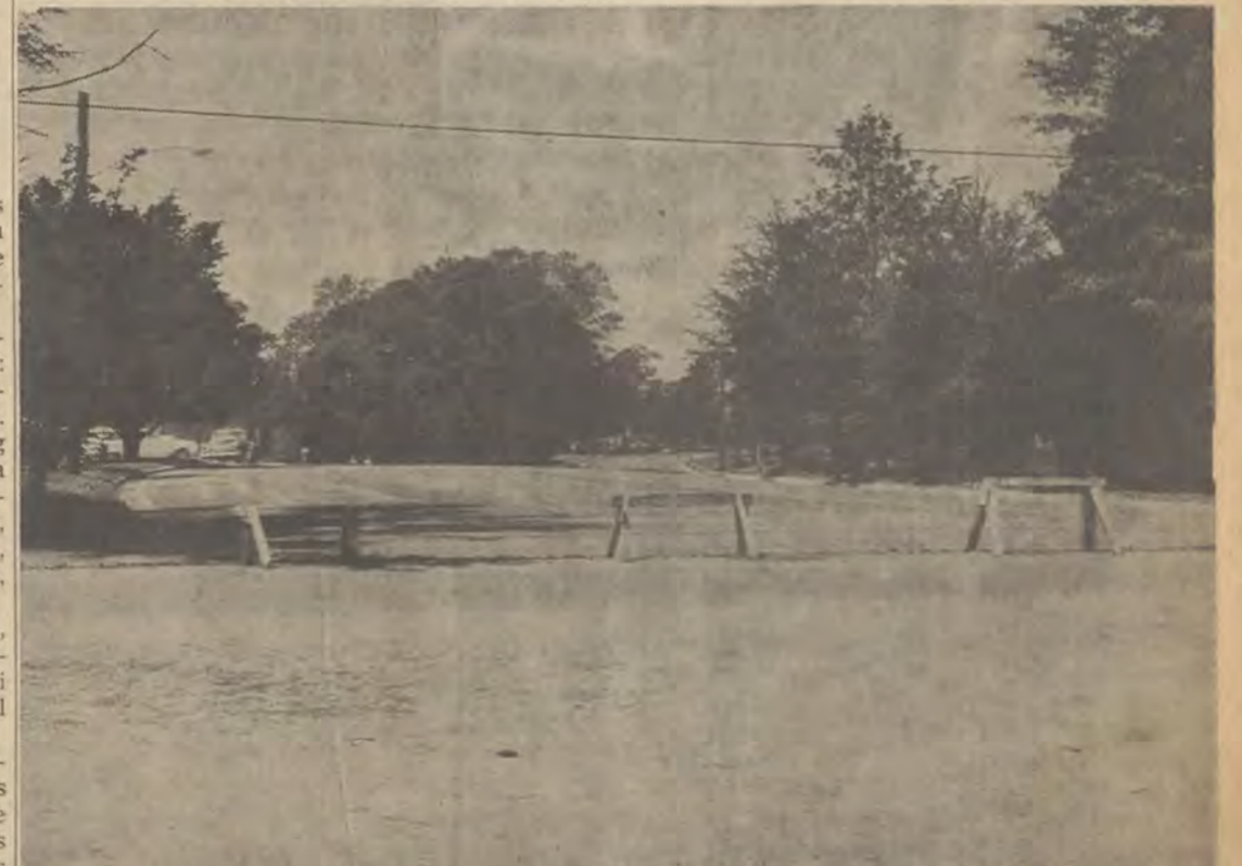
THIS IS A PICTURE of the road between the Frank I. Williams Center and the Carruth Building, which is being graded and paved for easier passage. The picture was taken during the lunch hour, which explains the absence of workmen in the area. No traffic is allowed to travel the road at the present time.
