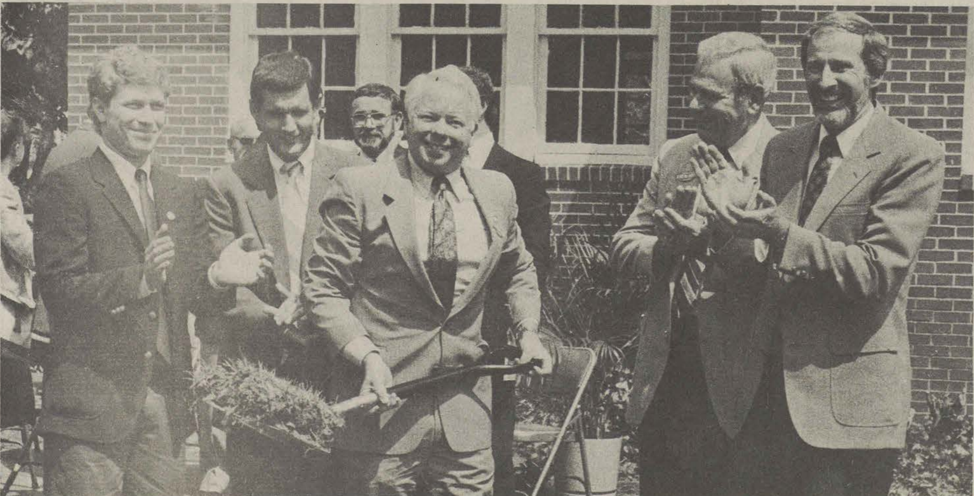
President Nicholas Henry is the first to "break ground" for the future $9.5 million Student Union Building scheduled for completion winter of 1989. (Photo by Frank Fortune)
