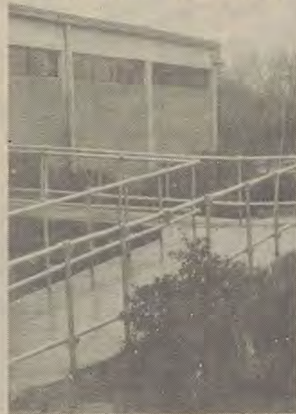
Handicap ramp at Landrum.
