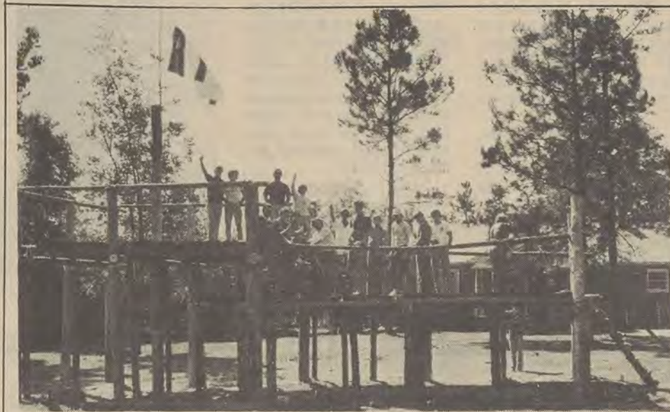
Several ATO Fraternity members stand on the structure they built for their Valhalla, (Viking Heaven) festivities which were held last weekend.
