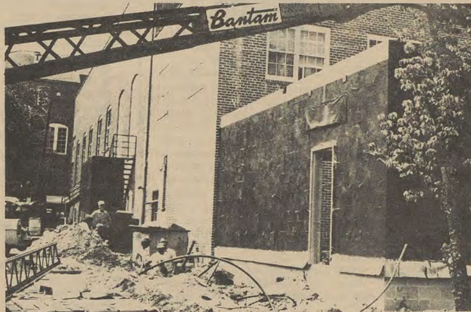
An annex was added to the rear of the Administration Building.
