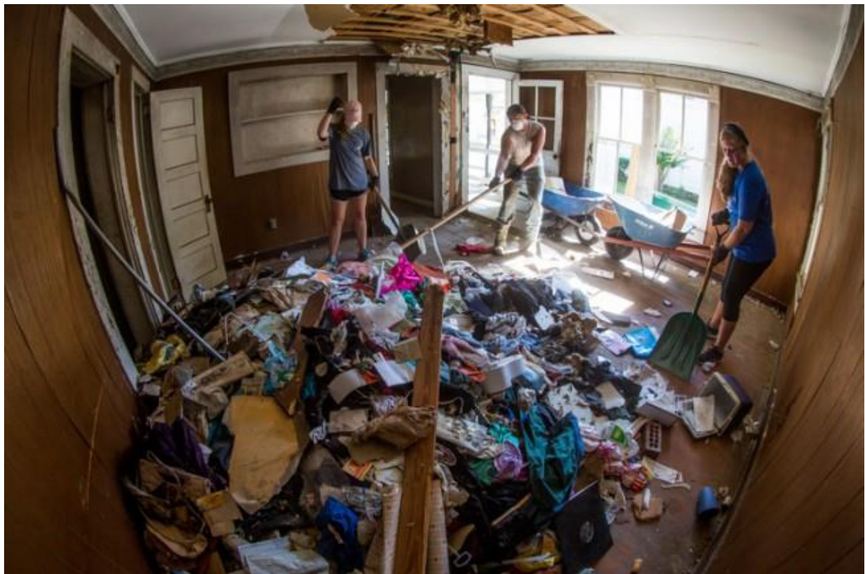
Student volunteers help clear an abandoned home to help the Downtown Statesboro Development Authority move forward with a renovation project.
