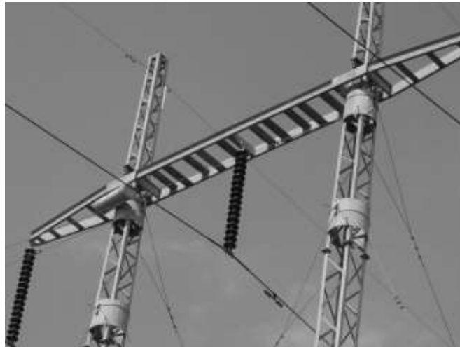
Figure 4. An example of the replacement lattice frame transmission tower containing no potential nest sites for American Kestrels.
