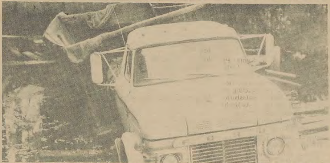
The 5,000 lb. maximum weight bridge on Groover's Mill Pond Road collapsed two weeks ago when an 8,000 lb. truck carrying 16,000 lbs. of
