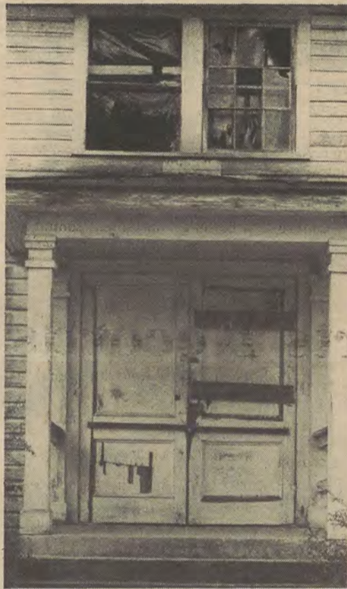
The entrance to one of Register's oldest schoolhouses. Weeds spurt from the dilapidated stairs and cracked plaster peels from weather-worn walls.
