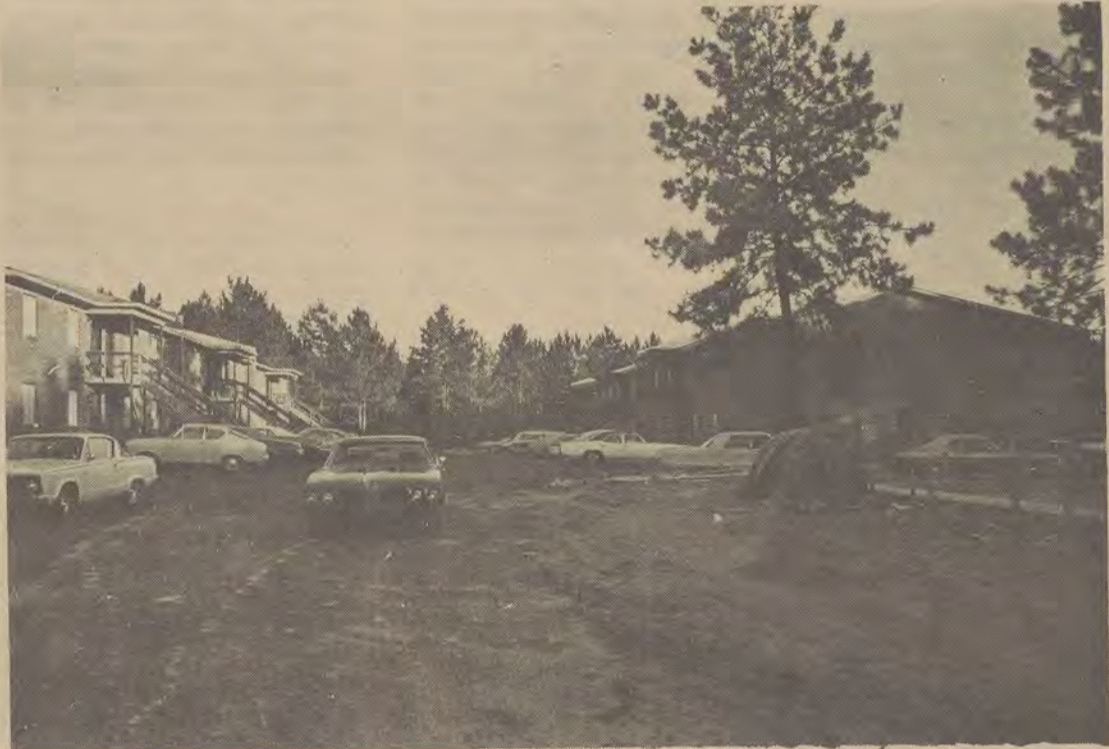
The new University City Apartments adjacent to the campus.
