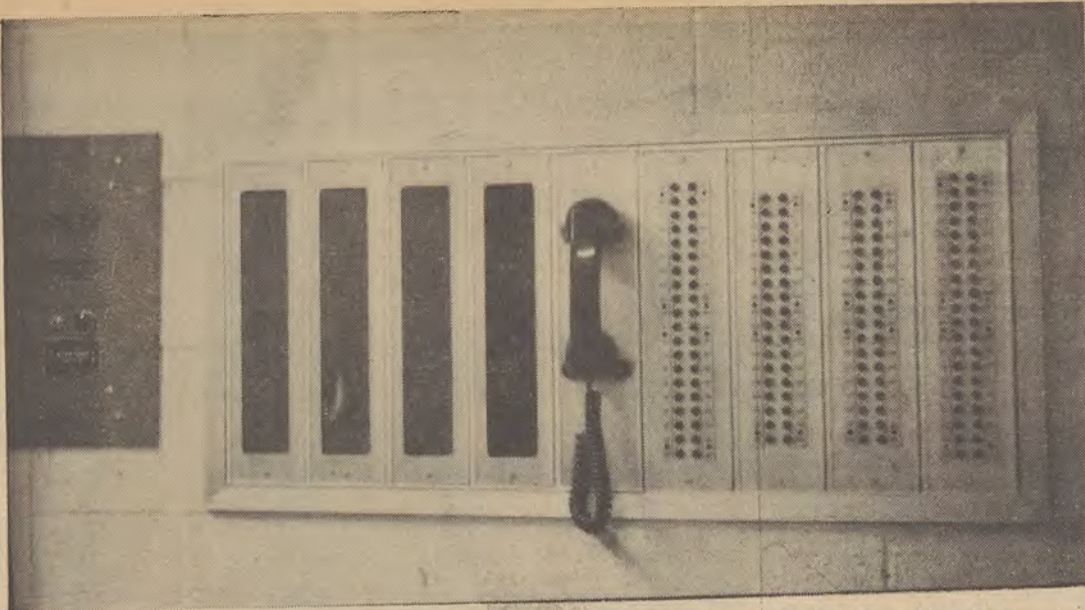
DORM HAS CONTROL BOARD FOR INTERCOM SYSTEM Each Room Features Individual Speaker Which Ties into Master Phone.
