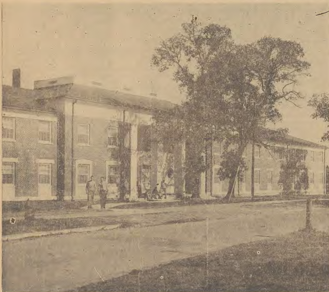
HOWELL CONE HALL—Recently completed men's dormitory at T. C. at a cost of $385,000, will be dedicated Saturday afternoon at 4 o'clock.
