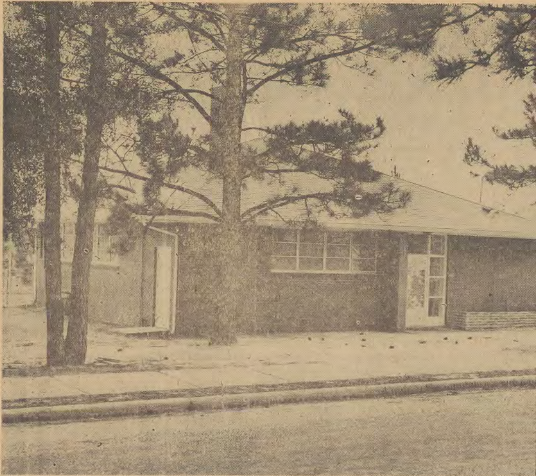
OUTWARD APPEARANCE of the recently constructed nursery building. The nursery was built in order that a home economic class, required under the university system could be taught at Teachers College.
