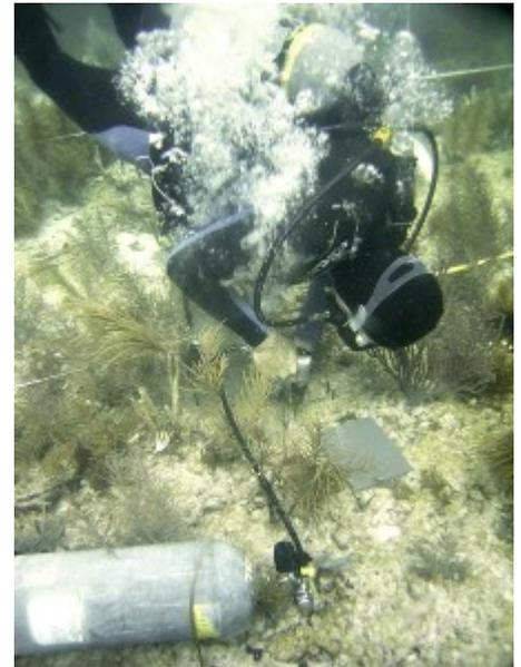
*Danny Gleason, Director, ICPS, uses a pneumatic drill connected to a scuba tank to create a small hole in the reef. A drywall anchor and stainless steel bolt will be installed in this hole.*
