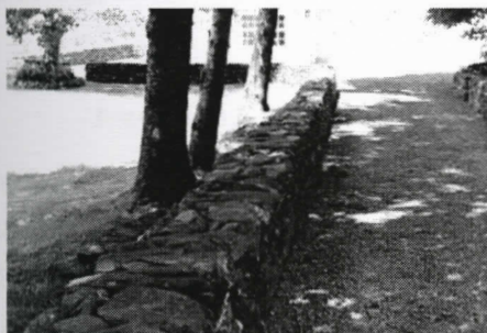
Figure 2. Traditional double-width dry stone construction
