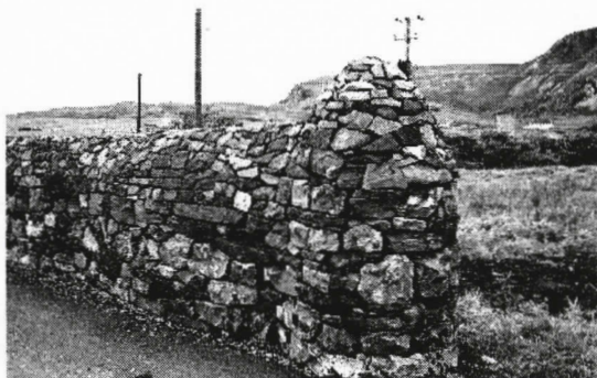
Figure 4. Fence built during dry stone construction training
