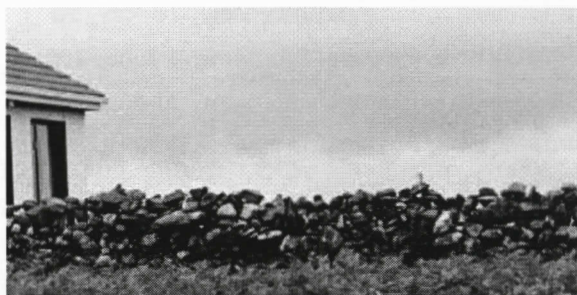
Figure 3. Traditional single-width dry stone construction. Note: Gapes in fence
