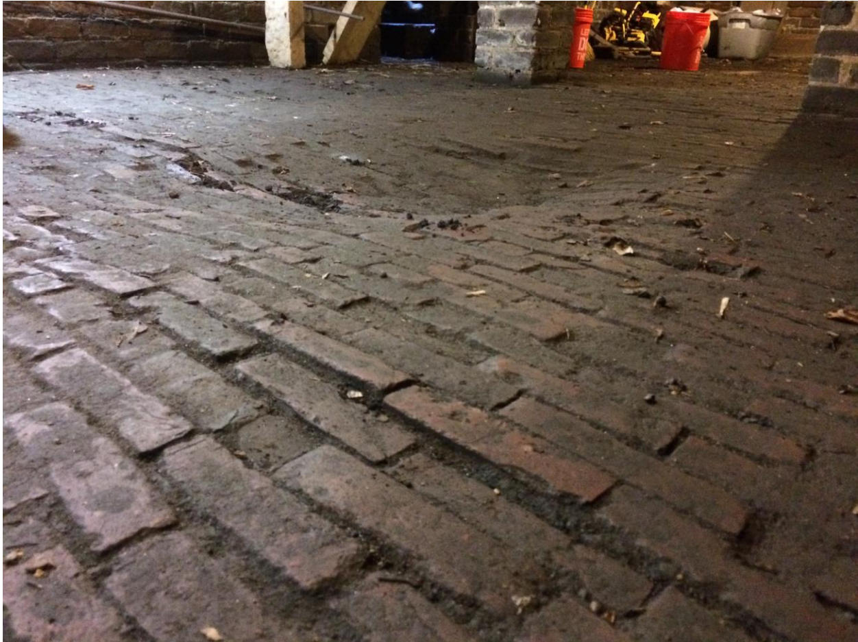
Depression in the floor of the carriage house basement at the Sorrel-Weed Home.
